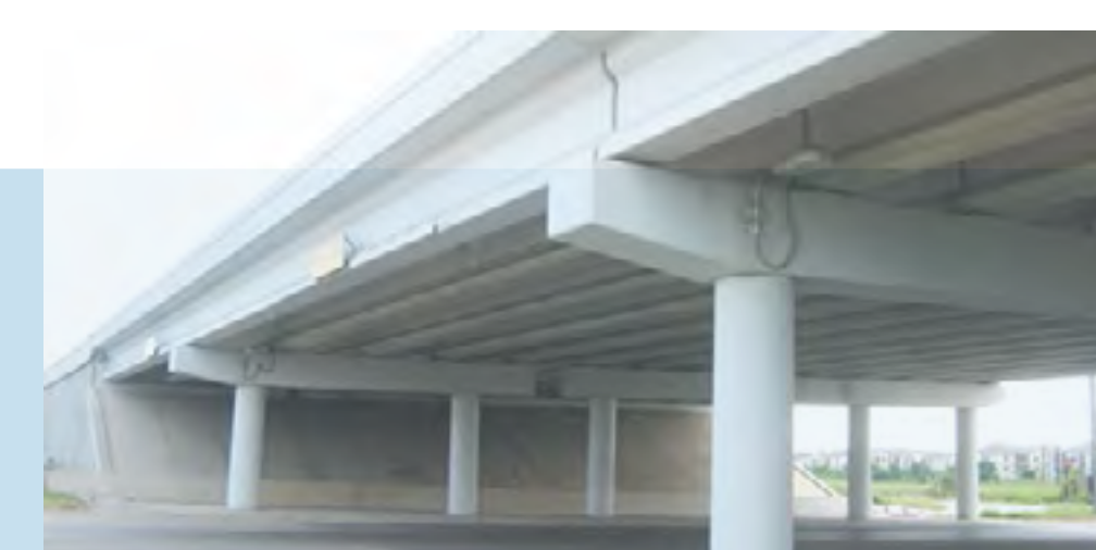
Bridge Enhancements: Existing Standard Construction 96 Respondents
