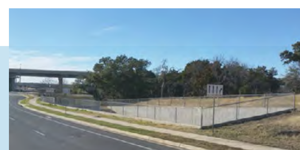
Water Quality Enhancements: Concrete Box Detention 134 Respondents
