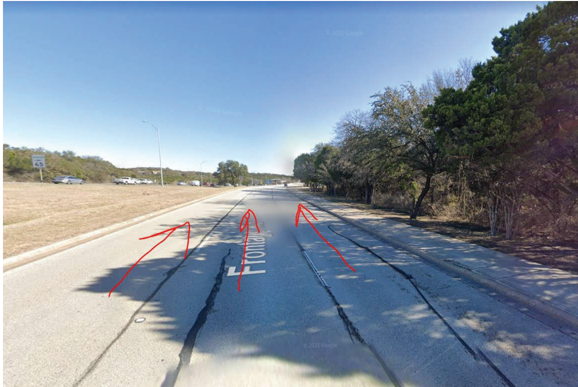
7. NB MOPAC frontage road has 3 lanes and a sidewalk.
