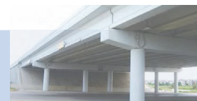
Bridge Enhancements: Existing Standard Construction 96 Respondents
