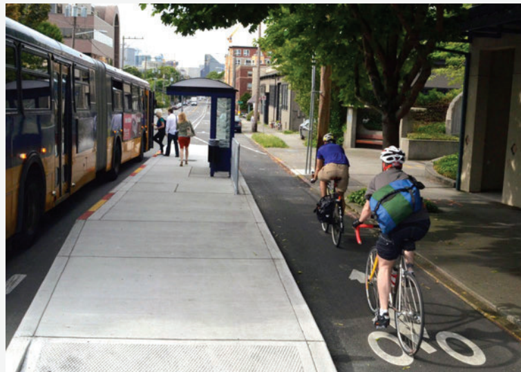
Figure 4. Transit island and bike lane in Seattle, WA. Photo by NACTO.
