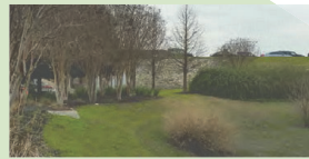
Water Quality Enhancements: Bio-Filtration Pond 131 Respondents
