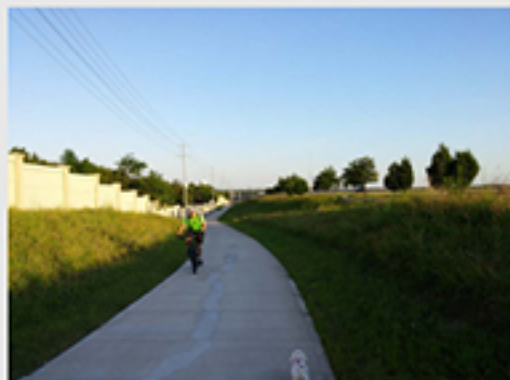
Shared use path along US 183A. Source: Jacobs 2015
